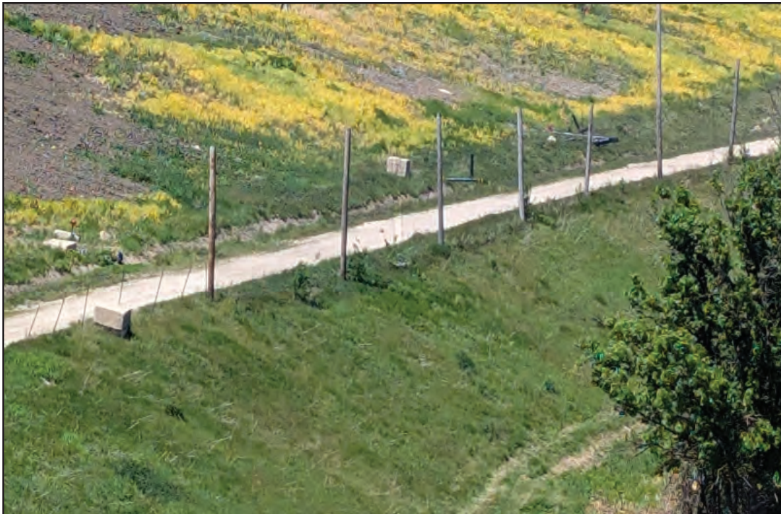
Post for tall fence being placed East of North Expansion West
