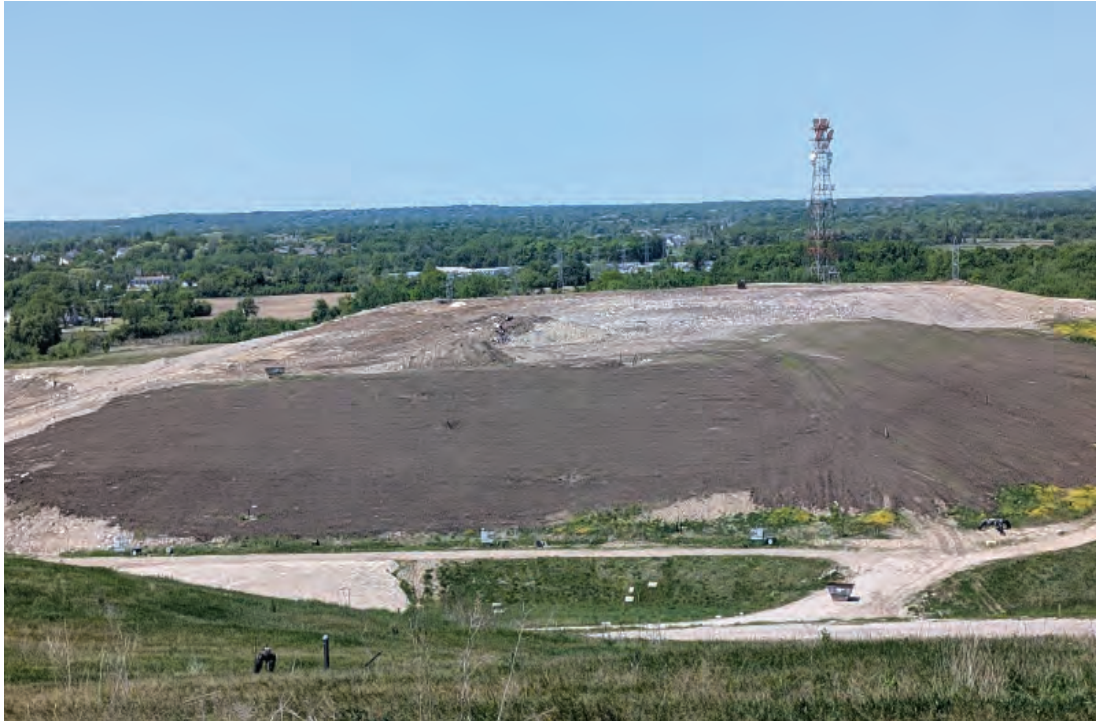
Top soil on North Expansion West, some vegetation starting to show
