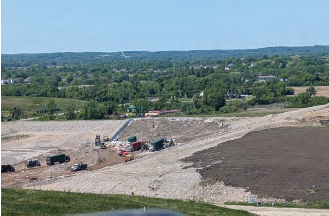
North end of Phase 4, current working face
