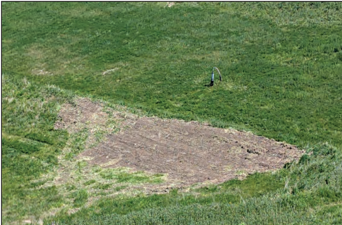
Erosion repair to berm on South slope of Phase 6
