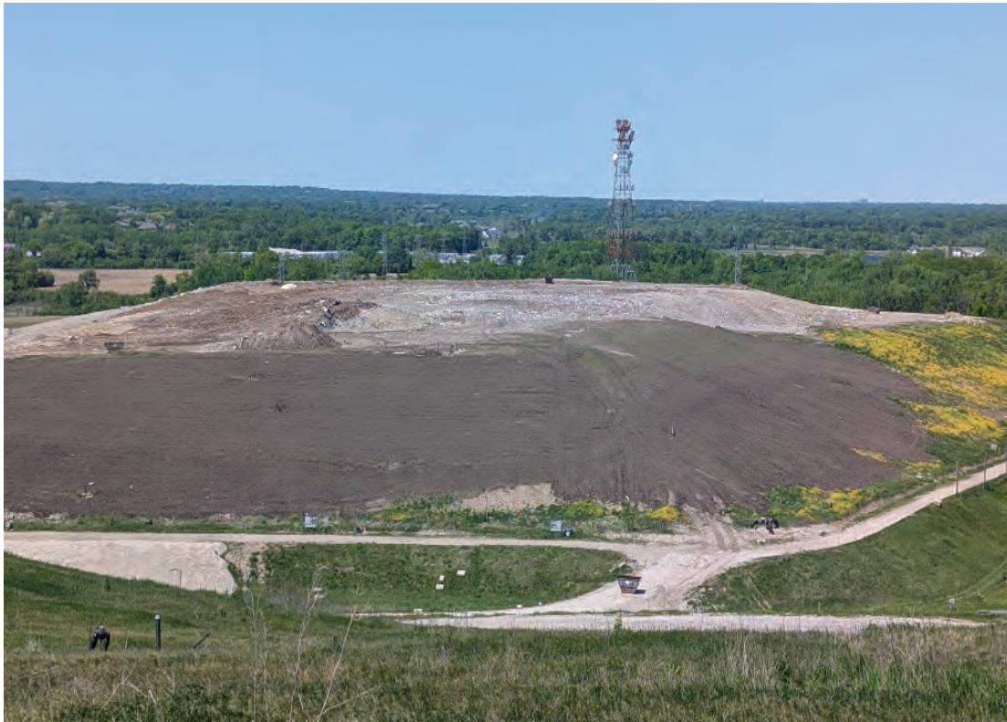
Top soil on North Expansion West; vegetation starting to show
